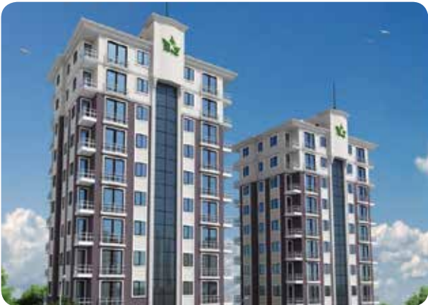
KARAMAN TOWERS, İSTANBUL
